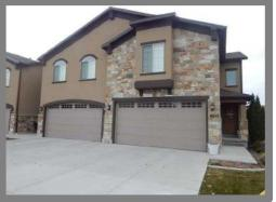
Concrete driveways on the property were generally in excellent shape as of the date of our review. Driveways are subject to wear with the constant freeze/thaw cycles occurring in this area. They are heavily salted and maintained during the winter months which also add to the wear in this climate. This component is the responsibility of the individual homeowners.
