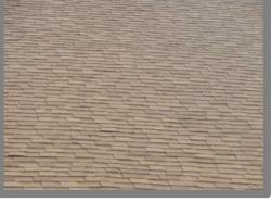
Roof is a 30yr architectural shingle which show no visible signs of wear. They are in new condition and there are no signs of damage throughout the property. Recommend full replacement after 27-30 years along with worn or damaged gutters and downspouts to take advantage of economies and ensure proper long term functionality.
