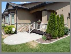
The stucco on the homes was in excellent condition at the time of our review. There were no visible cracks or water stress of any kind. The stucco is a two tone trim stucco with a 5" trim around all doors and windows on the property. Stucco in general requires regular maintenance and periodic repair as it ages. We recommend reserving for 7-10% damages every 3 years. This estimate will most likely increase as the property ages.
