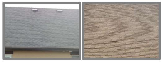
Roof is a 30yr architectural shingle which show no visible signs of wear. They are in new condition and there are no signs of damage throughout the property. Recommend full replacement after 27-30 years along with worn or damaged gutters and downspouts to take advantage of economies and ensure proper long term functionality.
